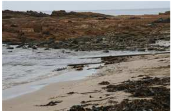
The existing boat ramp at Bastion Point, Mallacoota. (ABC Local: Catherine McAloon)
